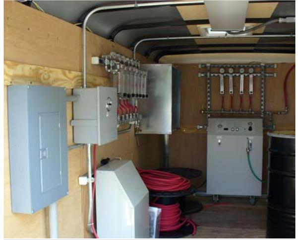
**Oxygen Generator<sup>®</sup>**: Oxygen generation for aerobic bioremediation systems. Oxygen generator uses the Pressure Swing Adsorption (PSA) process. It is the engine that drives the separation of oxygen from air. It is a purely physical process; there are no chemical, electrical, or other reactions in the process. 120 V power is required.
